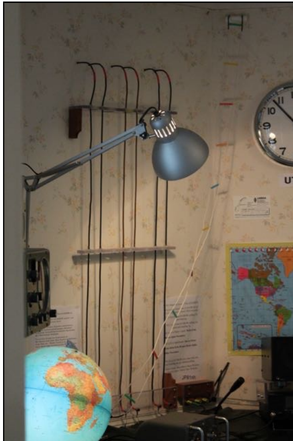
Spreaders inside the house are just tied with waxed twine.
