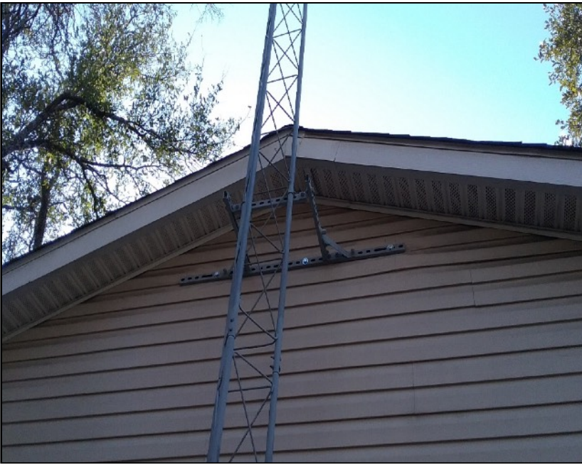
Rohn 25G attached to House via Home Brew House Bracket to tower
